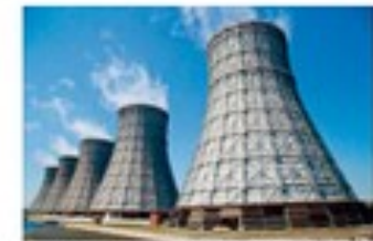
Figure 3: Cooling towers at a nuclear power plant. The steam used to drive the turbines is passed through the cooling tower to cool it down.
